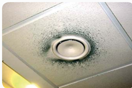
Fot. 1. Anemostat nawiewny zanieczyszczony cząstkami aerozolu ziarnistego i bioaerozoli Photo 1. Supply air diffuser contaminated by aerosol particle matter and bioaerosols
